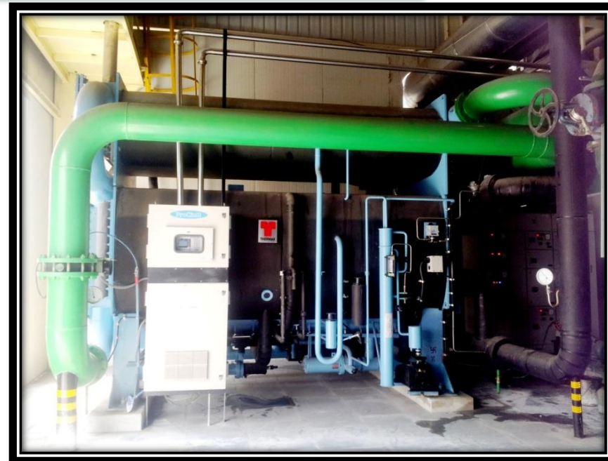
Chiller Capacity : 680 TR at Pepsico
